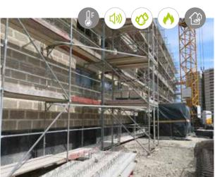
**Project:** New build of a commercial building in 30cm hemp blocks and load-bearing structure of concrete blocks. For use as a logistics centre and numerous offices.
