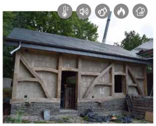
**Project:** New build of a detached home with a timber columns-beams structure and hemp blocks of 20cm and 30cm. Low energy house with exterior facing of stones attached directly to the insulating block.
