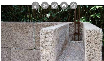
**Project:** New build implemented with the IsoHemp Hempro system. Construction system comprising concrete columns-beams poured directly into 30cm hemp blocks. A supplementary envelope of 20cm thickness was built to achieve a home meeting the passive building standard.
