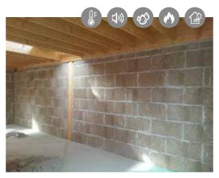
**Project:** New build of two very low energy houses with a timber column-beam structure with a complete single wall outer envelope of 42cm made from hemp blocks (12cm + 30cm). Lime render exterior finish.
