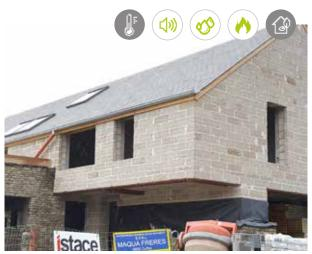
**Project:** New build in 30cm hemp blocks laid in the envelope of load-bearing concrete blockwork. The client wanted a strong and insulating substrate for application of the exterior finishes. He chose hemp blocks for application of a lime-based render and attachment of the facing stones directly to the insulating block without creating any thermal bridging.
