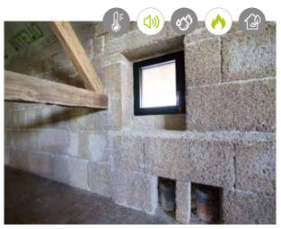
**Project:** Renovation of an old half-timbered farmhouse with hemp blocks. A complete interior envelope was built using 15cm hemp blocks. This solution avoids any potential condensation problem or degradation of the timber frame.
