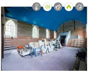
**Project:** Low energy renovation of an old church. Interior insulation provided by 30cm hemp blocks. Wall heating and interior clay-based finish.
