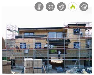
**Project:** New build of an apartment block make of CLT timber with 30cm hemp blocks for the outer envelope. The client wanted natural breathable insulation. The interior partitions were all made using 12cm hemp blocks to improve the acoustics of the living spaces.
