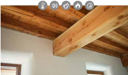
**Project:** New build of a detached house. Combination of a formwork of hemp concrete and hemp blocks. Load-bearing columns-beams structure and timber framework. Interior and exterior lime-based finishes.
