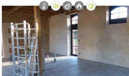
**Project:** Interior renovation and restoration of an old farmhouse (previously a pig farm) using 20cm hemp blocks. Preservation of the external look of the building in authentic old stones. Application of an interior lime-based plaster.
