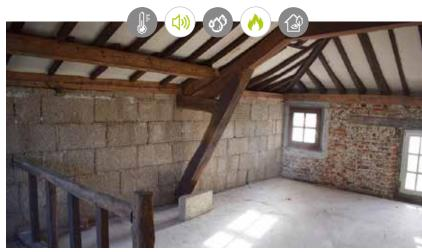
**Project:** Complete interior renovation of an old barn using 15cm hemp blocks. Preservation of the inner look as well as the original frame while avoiding any potential condensation problems or degradation of the wooden framework. Interior finishing with natural lime-based plasters.
