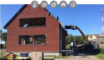
**Project:** Building of a very low energy detached house with a metal load-bearing structure and complete 30cm + 9cm hemp block envelope with an exterior finish of facing bricks. Selection of an economic structure that can be quickly installed, without compromising the efficient performance of the building envelope.
