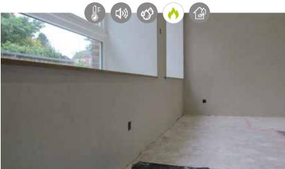
**Project:** Interior renovation using 20cm hemp blocks of a school and classrooms. Interior finishing performed using IsoHemp's PCS natural interior plaster coating. The thermal and sound insulation of the brick building was considerably improved.
