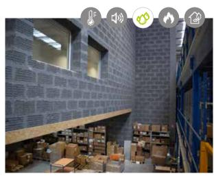
**Project:** Construction of blockwork, 30cm x 25 metres wide x 14 meters high forming a division between heated offices and a storage area. This unique blockwork provides simultaneous thermal and sound insulation of the two spaces while complying with fire safety standards. The blockwork was plastered on one side and spray painted on the other to achieve optimum sound absorption.
